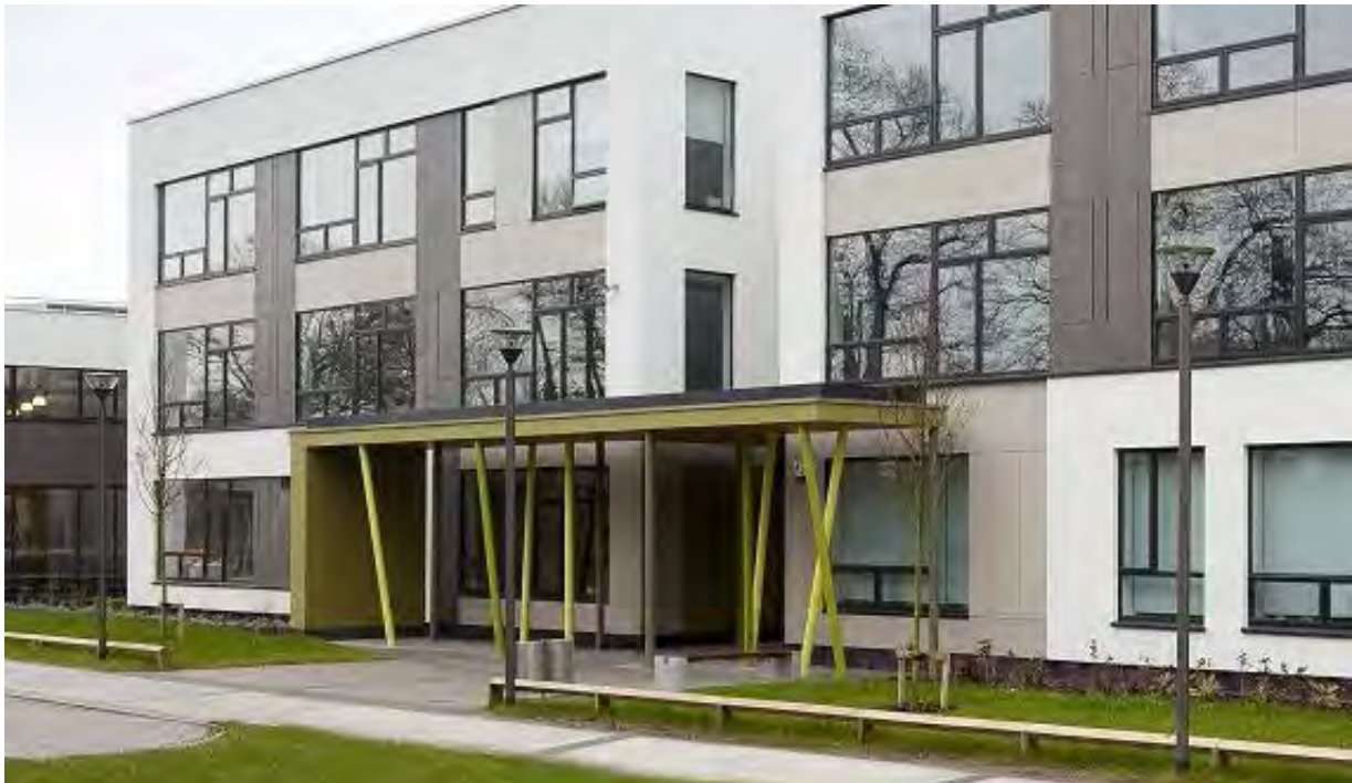
Figure 3 - Coláiste Choilm in Tullamore which won the SEAI Energy Sustainability in the Built Environment Award for 2012 (Photo by Donal Murphy www.donalmurphyphoto.com )
