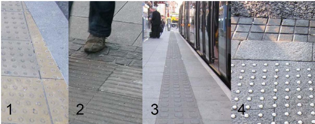
Figure 2.2: Typical tactile paving types
