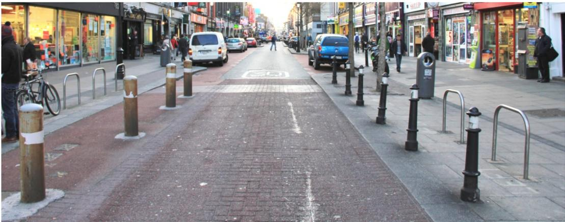
Figure 12.9: Raised traffic islands like the one pictured here provide a level crossing, a narrowing of the carriageway and an crossing point where drivers typically give way to pedestrians crossing. This functions in a similar way to the courtesy crossing discussed here.
