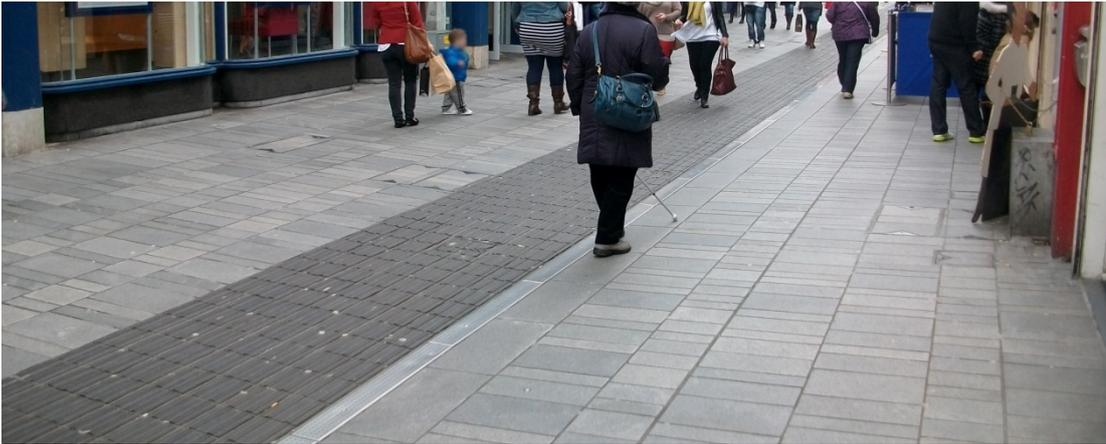
Figure 12.10. Example of a tactile strip as a way-finding device
