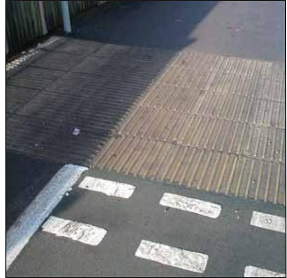
Where used to warn of an approaching flight of steps, corduroy paving should extend to the full width of the steps, plus at least 400mm to either side wherever possible. However, the corduroy paving must not extend across an adjacent ramp, access route or facility such as a lift.
