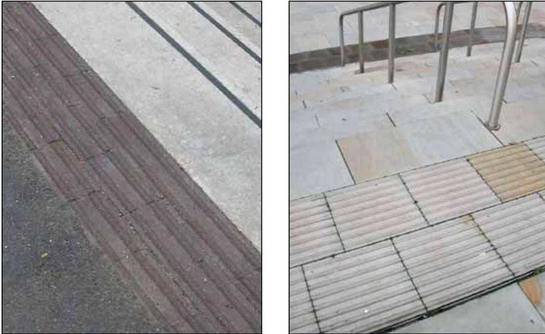
Hazard Warning units use continuous half-rods, raised 6mm higher than the surface of the paving, to denote a hazard, such as the top/bottom of a flight of steps. Again, the rods should be parallel to the edge of the hazard.
