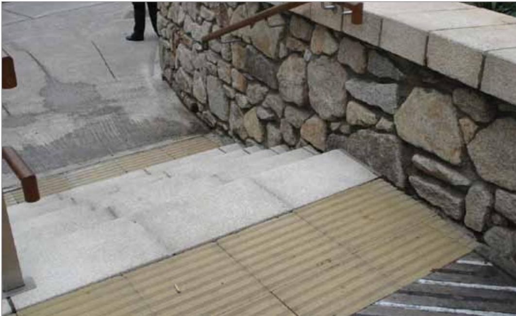
The hazard warning surface should be positioned sufficiently in advance of the steps to give adequate time to stop. It should also extend a sufficient distance in the direction of travel to ensure it is detectable to all pedestrians. If only a narrow strip is provided, a person may step over it with a single stride and be unaware of the approaching hazard. The location and dimensions of hazard warning surfacing for external steps are illustrated in **Figure 1.13**.
