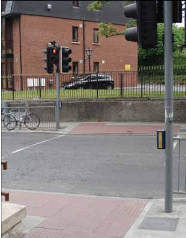
**Image 1.37b and Image 1.37c** Example red blister paving.
