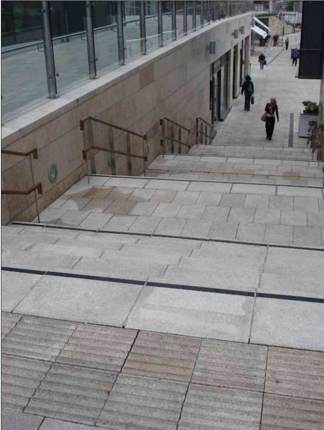
Steps can present a hazard to people with visual difficulties, particularly when they are located in the direct line of travel. The use of a tactile hazard warning surface at the top and bottom of a flight of steps provides a means of highlighting the approaching change in level. However, it must be of the appropriate type and be installed correctly in order to convey the right message and to provide adequate warning to pedestrians.
