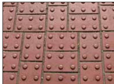
The Offset Blister units are used to indicate the edge of the platform at Rail and Tram stations, also referred to as off-street applications. Note that the orientation of the offset blister units is critical - the rows of blisters **MUST** be parallel to the platform edge, and they are generally placed approximately 500mm back from the edge.
