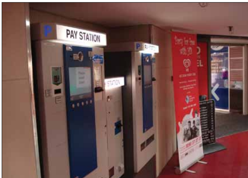
Image 1.18 Example of car park ticket pay stations with different heights of ticket slot.
