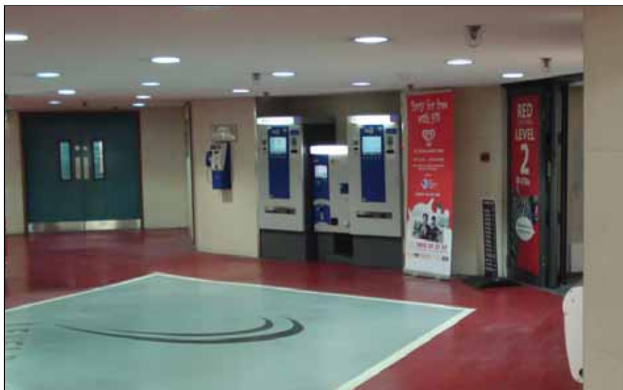
Image 1.21 Example of ticket machines located within easy access of entrance to and from the car park.
