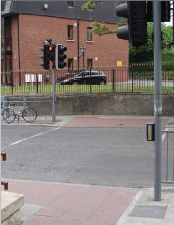
Image 1.37a Example red blister paving.
