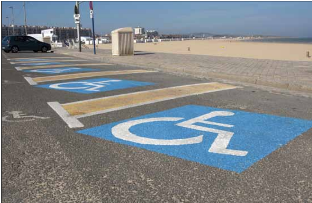
Image 1.4 Example of insufficient accessible parking spaces. Please note the lack of a post-mounted sign with the international symbol of access fixed to it and the lack of dropped kerbs.
