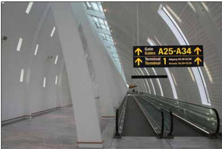
Image 3.26 Example of travelator with emergency stop button and guard rails alongside pedestrian corridor.
