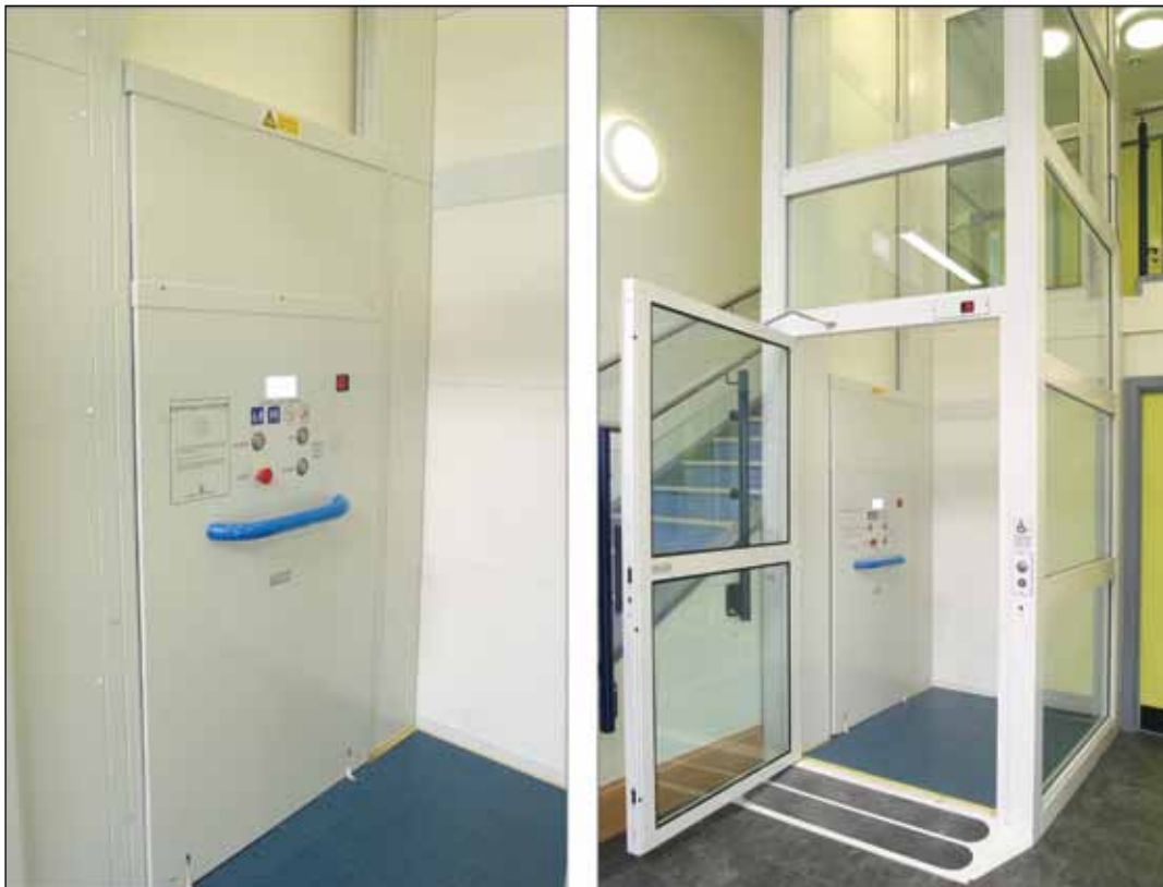
Image 3.13 Example of vertical platform lift showing interior and controls of lift.
