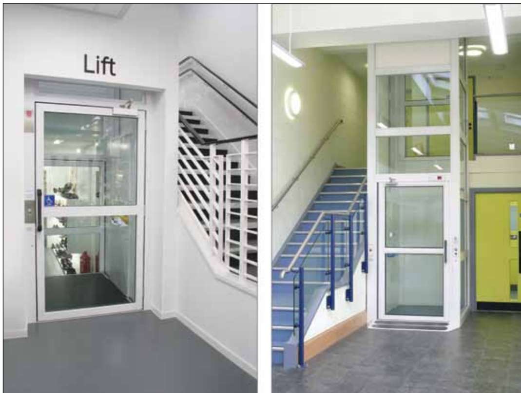
Image 3.12 Example of a vertical platform lift with an associated flight of steps.
