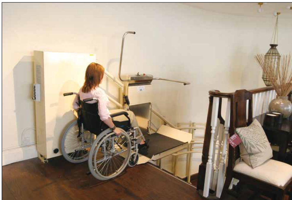
Image 3.16 Example of an inclined platform stairlift.
