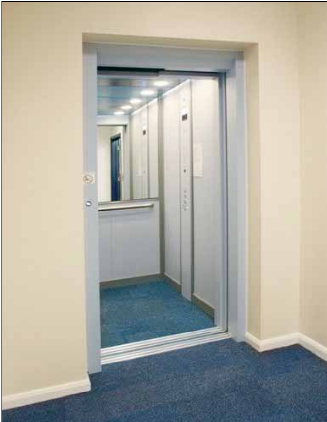
Image 3.9 Example of lift with contrasting floor and walls. Also note the mirror and grabrail on the wall opposite the door.
