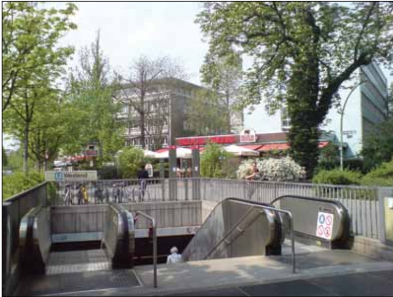
Image 3.23 Example of external escalator showing tactile hazard warning strips on both up and down directions.
