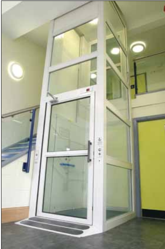
Image 3.11 Example of a vertical platform lift.
