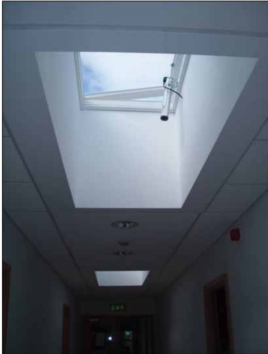
Image 4.8 Example of natural light used to light a corridor.
