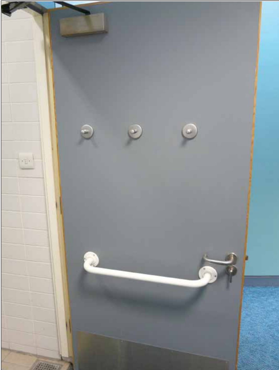
Image 5.3 Example of door-mounted grabrail.
