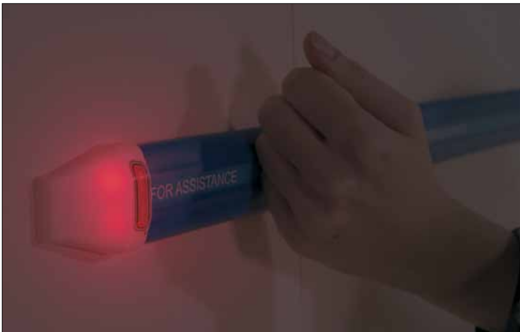
Image 5.25 Alternative view of the dado level panic strip in use.
