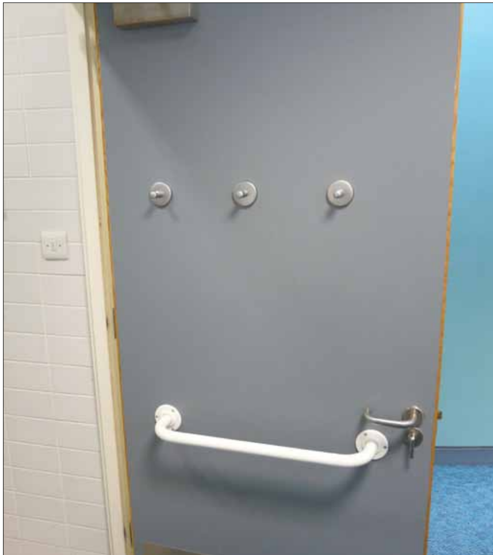
Image 5.29 Example of door-mounted grabrail.
