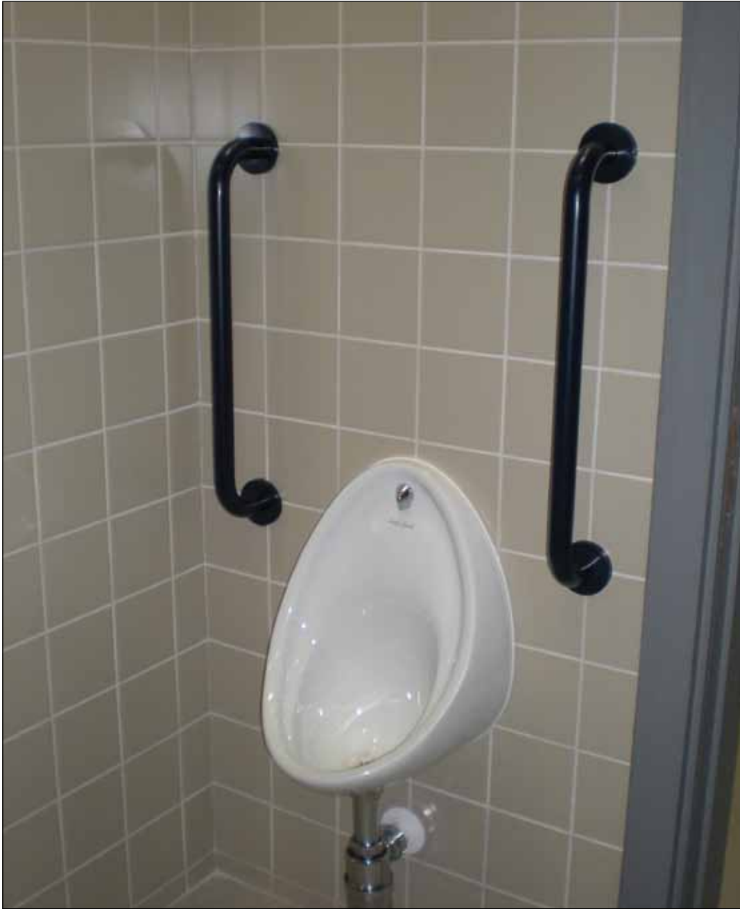
Image 5.6 Example of accessible urinal with grabrails.
