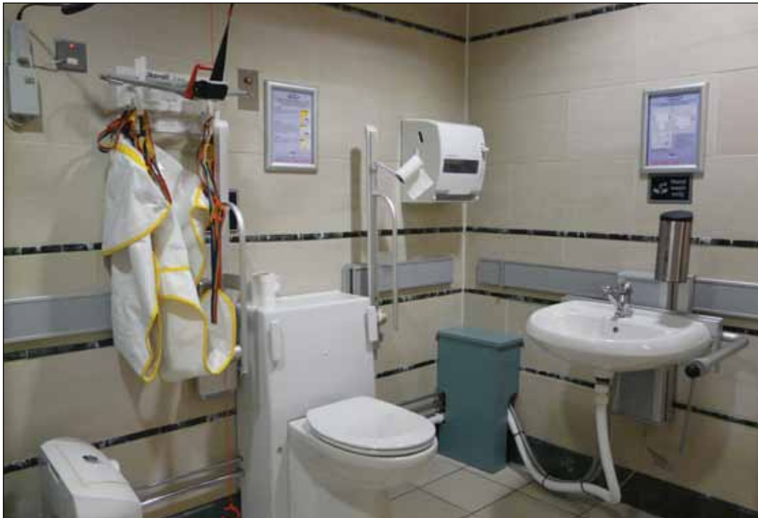
Image 5.16 Example of unisex peninsular-arrangement toilet with assisted changing.
