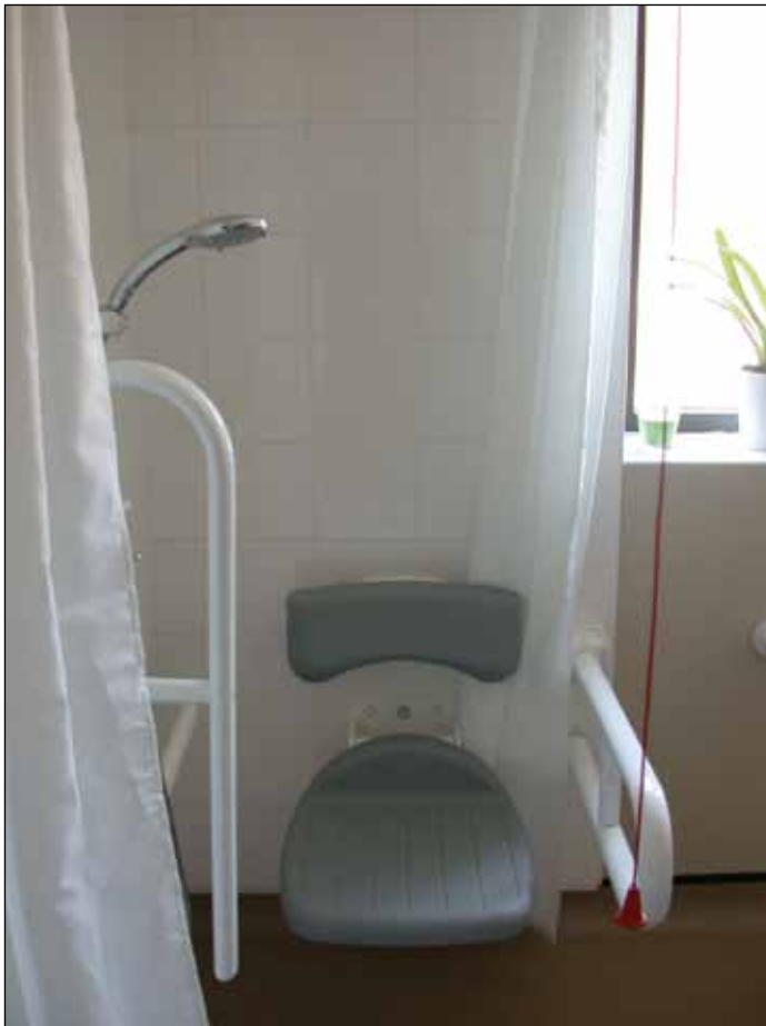
Image 5.20 Example of a fold-down shower seat.
