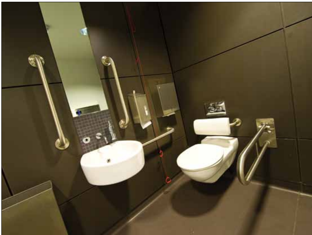
Image 5.10 Example of unisex accessible toilet – Right-handed transfer.
