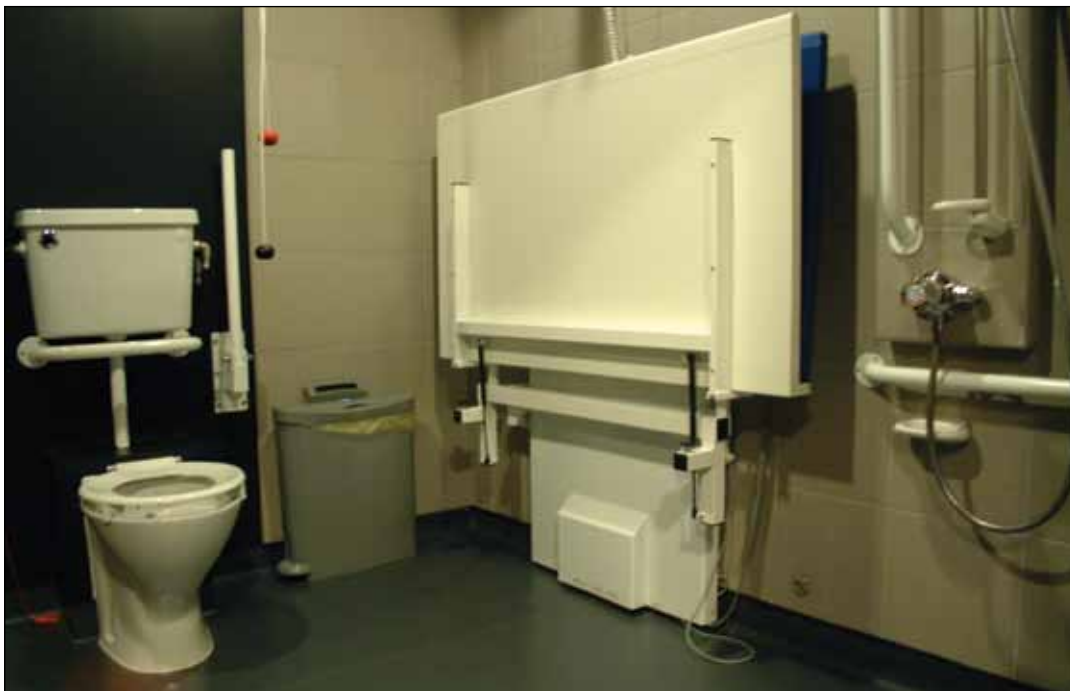
Image 5.16 Example of unisex peninsular-arrangement toilet with assisted changing.
