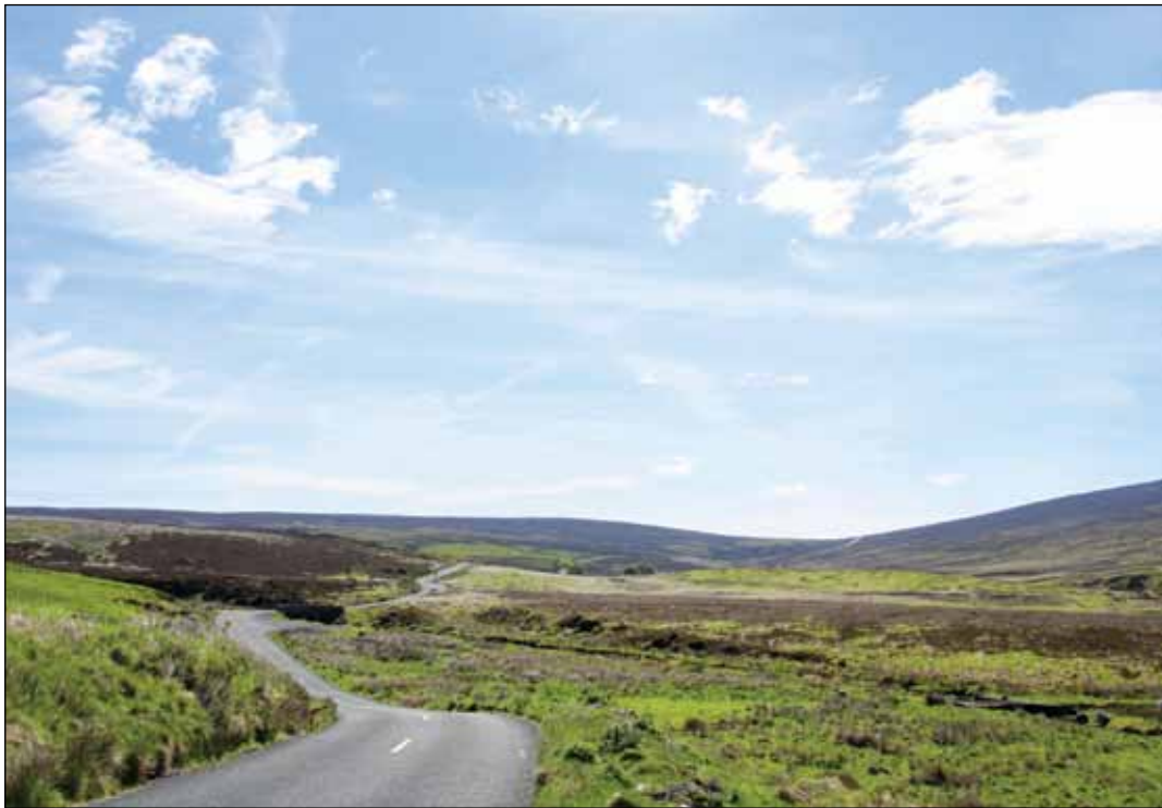
Image 7.24 Example of peatland with a road running through it.
