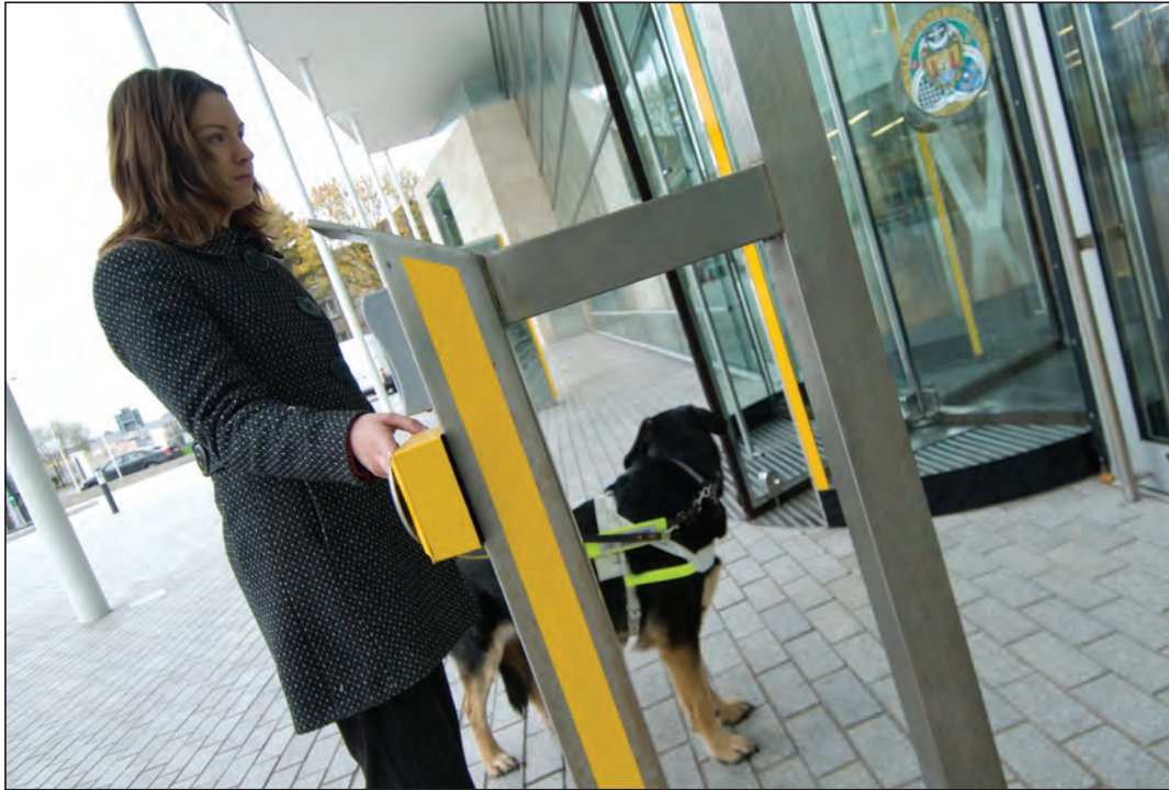
Image 2.30 Example of powered door with push plate.
