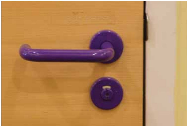
Image 5.27 Example of a lever door handle.
