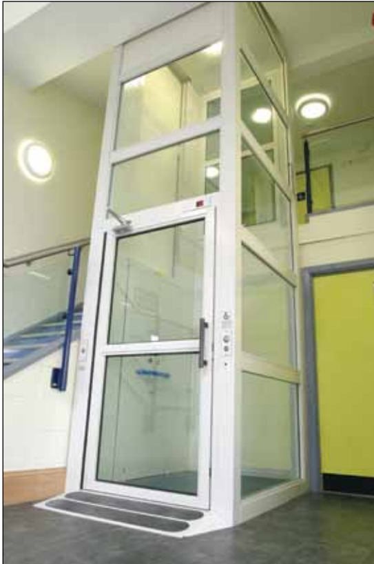
Image 3.11 Example of a vertical platform lift.
