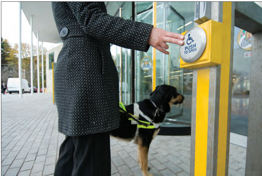
Image 2.29 Example of powered door with push plate.
