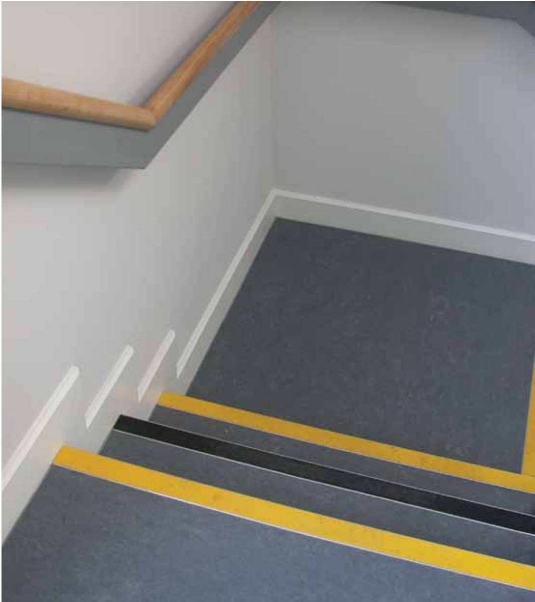
Image 3.1 Example of stairs with non-slip applied nosing.
