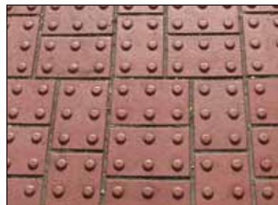
Image 1.37b and Image 1.37c Example red blister paving.
