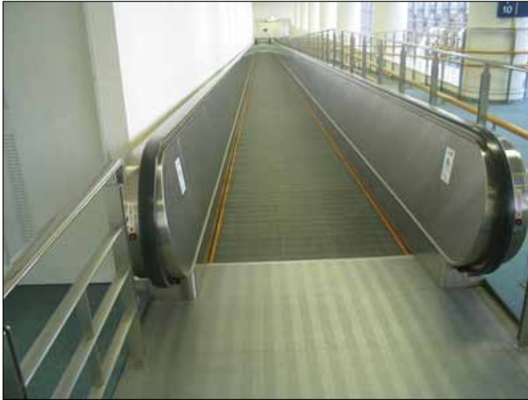
Image 3.24 Example of inclined travelator.
