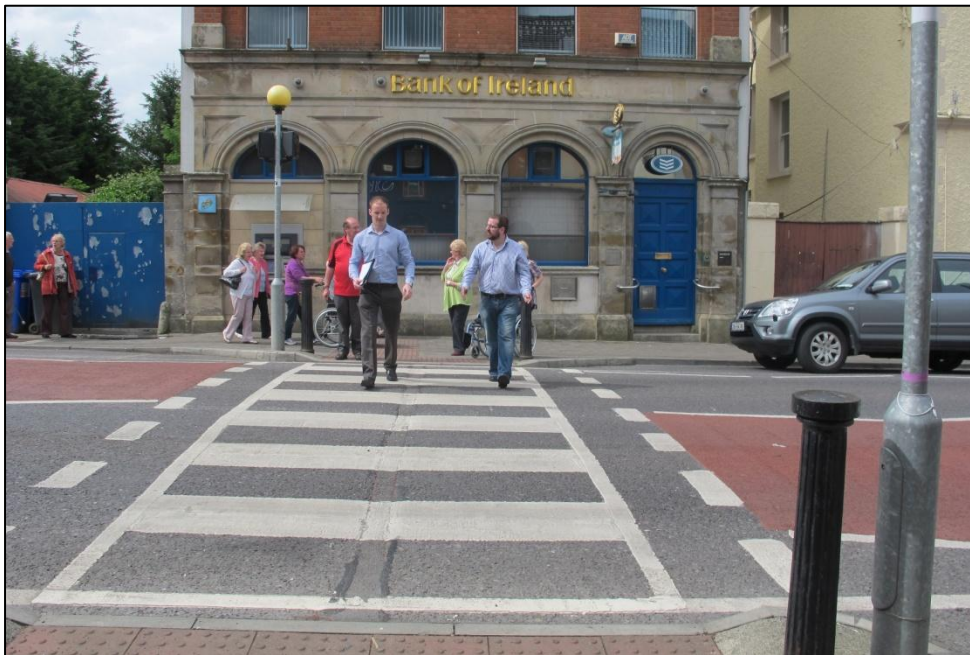
Image 3.1 An example of a zebra crossing with dished kerb and tactile paving.
