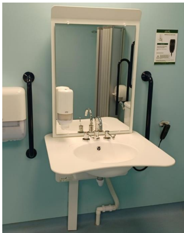
Image 9 - Example of a washbasin that can change height, from Kildare County Council
