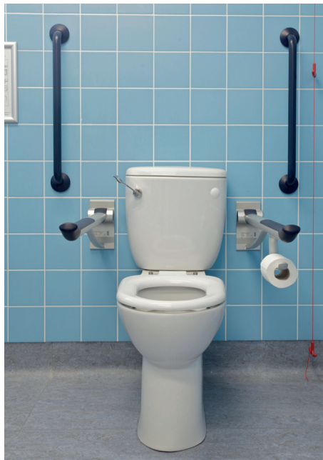
Image 3 Wheelchair Accessible Unisex WC with corner WC pan arrangement and washbasin within reach of the WC pan
