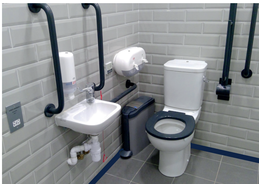
Image 3 Wheelchair Accessible Unisex WC with corner WC pan arrangement and washbasin within reach of the WC pan
