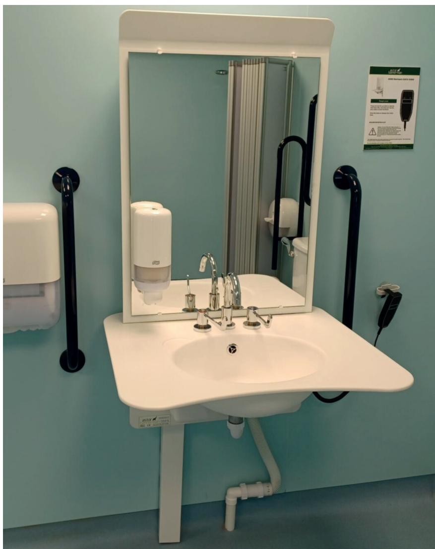
Image 9 Example of a height-adjustable washbasin, courtesy of Kildare County Council
