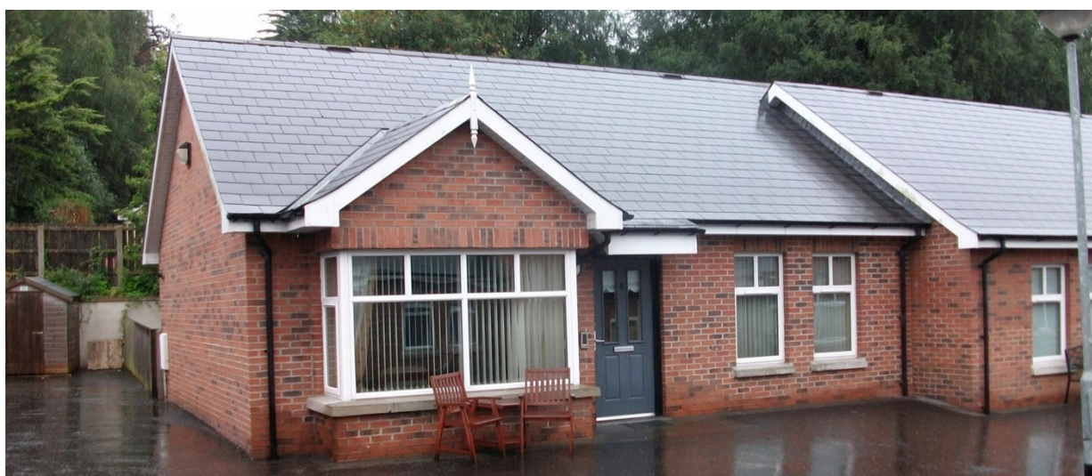
Figure 34 – View to the front entrance of a typical bungalow
