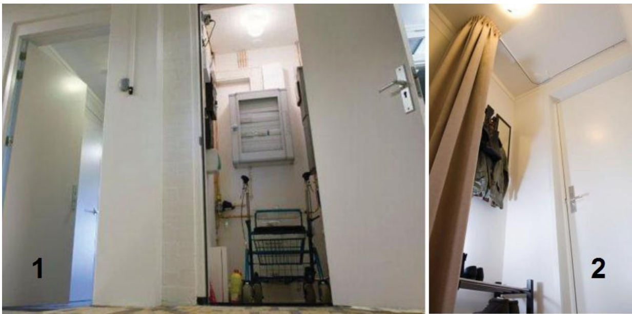
Figure 13- Image 1 shows a services cupboard in the common hallway external to the dwelling. Image 2 shows a curtain that can be drawn across the internal face of a door to hide the exit.
