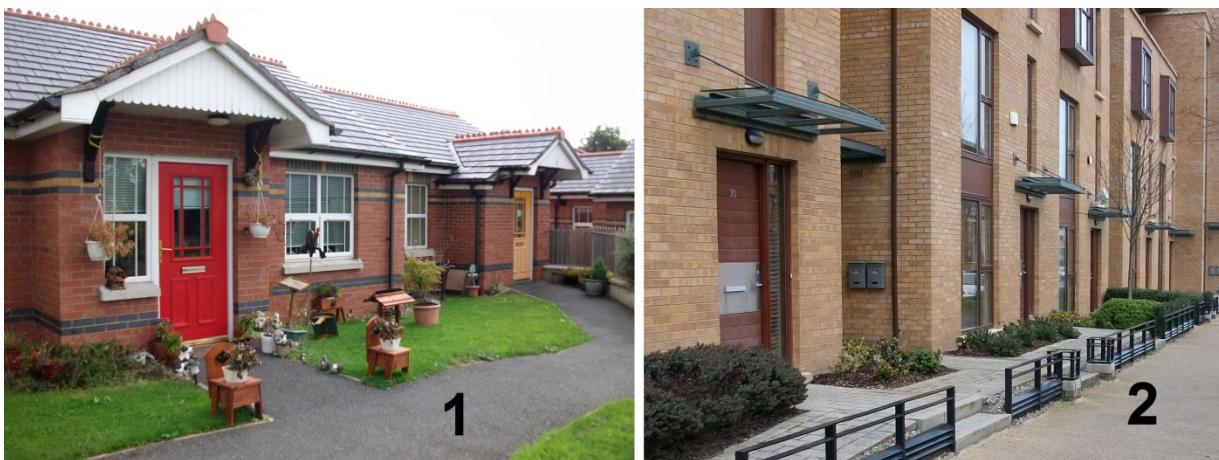
Figure 11 - A traditional entrance canopy and a contemporary canopy
