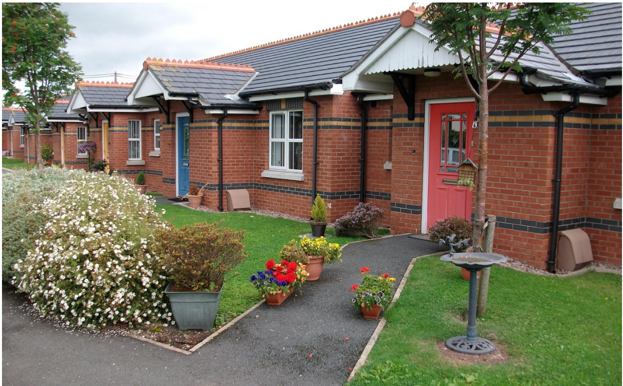
Figure 29 – Exterior view of Barn Halt Cottages, Carrickfergus, Co. Antrim
