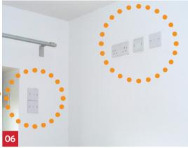
Data and power connections are provided at 2300mm for future assisted living technologies installations, and adjacent to windows for actuators.
