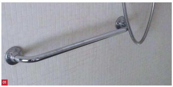
A strong load bearing surface has been provided throughout the shower room to allow for firm fixing of handrails wherever they might be required.
