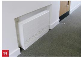
A low surface temperature radiator is recessed into a wall to avoid creating an obstruction and narrowing the corridor. There is no colour contrast between the wall and radiator which might make it difficult for some people to locate.
