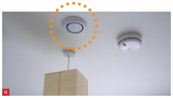
A vent is provided in each room to supply a constant flow of fresh pre-heated air. Stale and moist air from bathrooms and kitchens is extracted.
