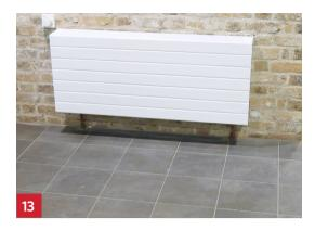
A low surface temperature radiator is provided with the TRV control between 450 and 1200mm above floor level. There is good colour contrast between floor, wall, thermostatic radiator valve (TRV) control and radiator.
