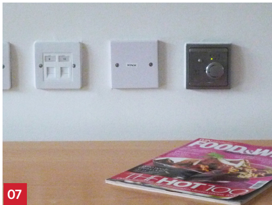
07 Sockets are provided at a consistent height and level.
