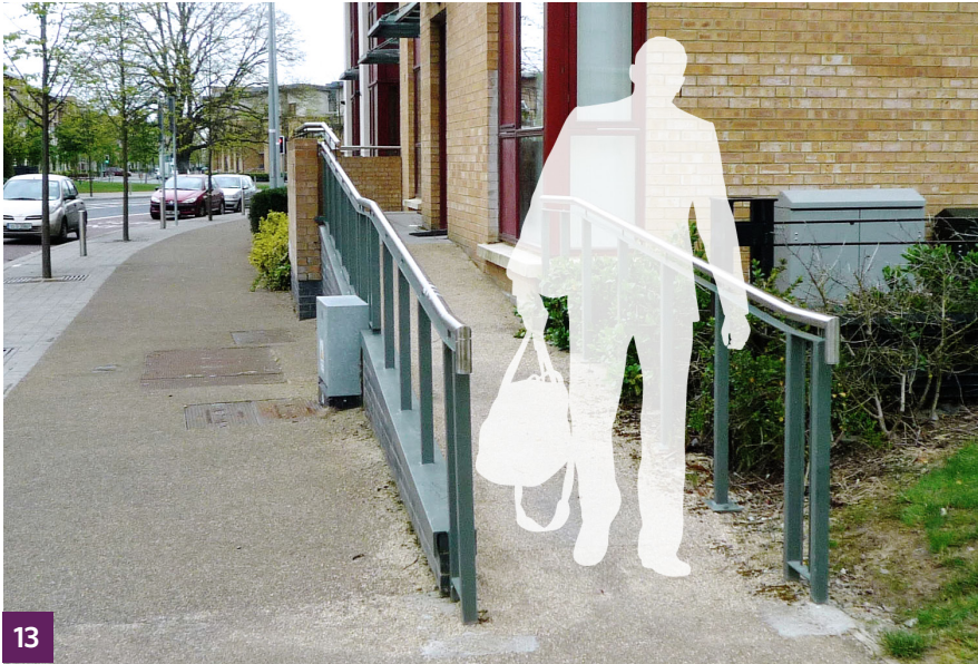
Ramp and landings provided to raised ground floor with handrails on both sides.
