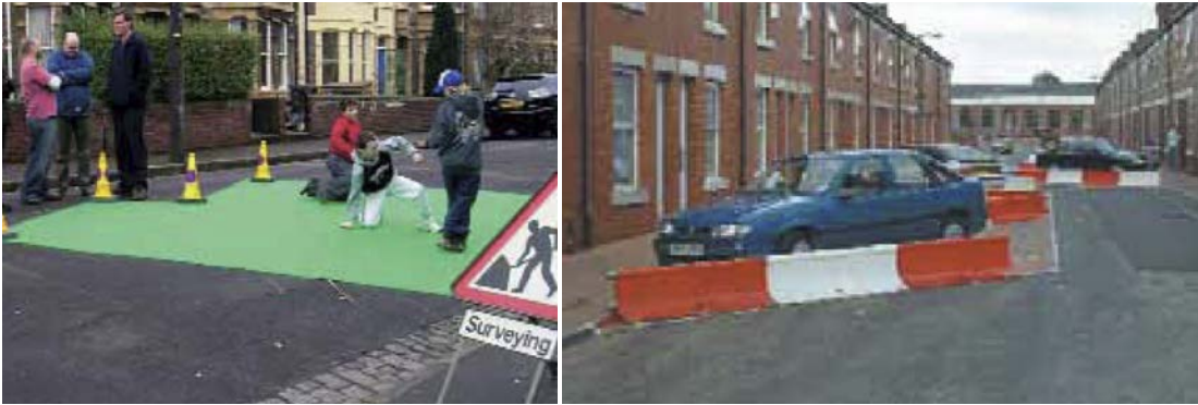
Figure 12.1: On street mock-ups to represent proposed changes to street design (Department for Transport UK, 2005a)
