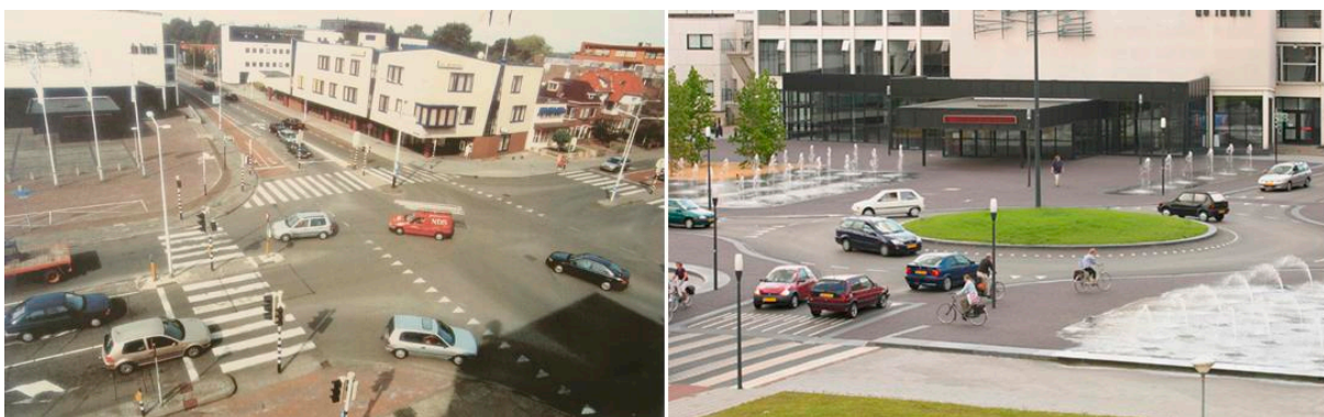
Figure 3.12 – Laweiplein junction Drachten before and after Shared Space design measures were implemented (Hamilton-Baillie, 2008b)
