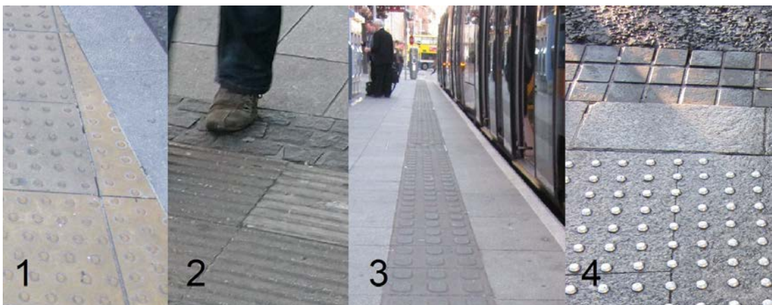
Figure 12.4: Typical tactile paving types. 1 – blister paving, 2 – corduroy paving, 3 – warning paving and 4 – metal stud blister paving. (long description to be included)
