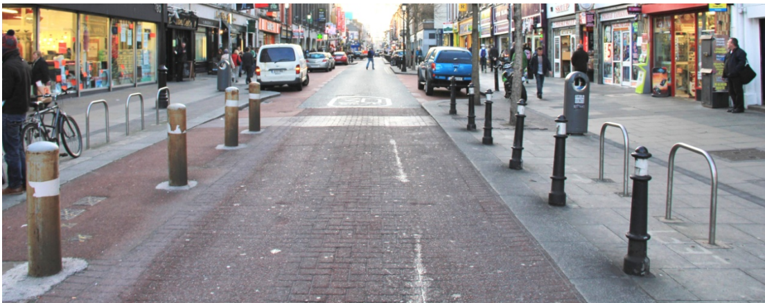
Figure 12.9: Raised traffic islands like the one pictured here provide a level crossing, a narrowing of the carriageway and an crossing point where drivers typically give way to pedestrians crossing. This functions in a similar way to the courtesy crossing discussed here.
