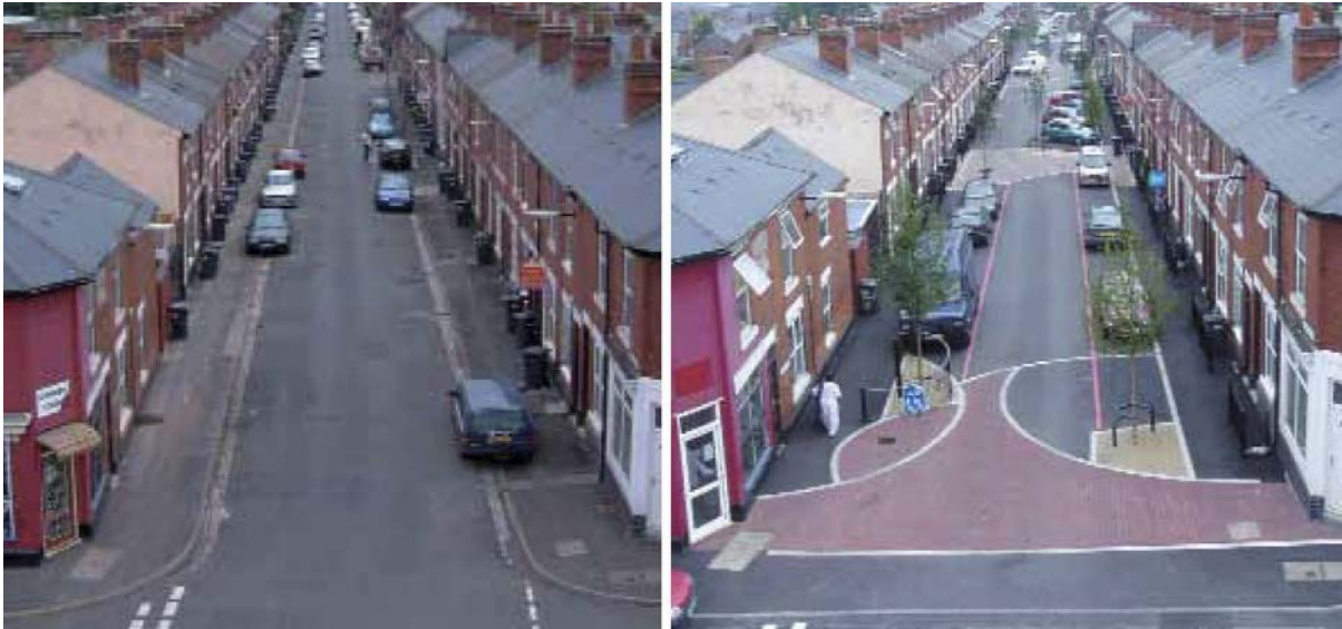
Figure 3.19 – Before and after photographs of a street in the UK redesigned as a Home Zone (Department for Transport UK, 2005a)
