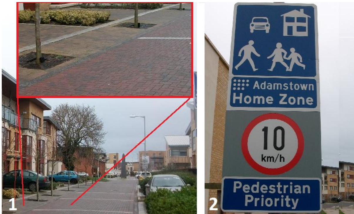
Figure 9.9 – Design features of Castlegate Down Home Zone. Image 1 – Shared Surface. Image 2 – Home Zone signage.
