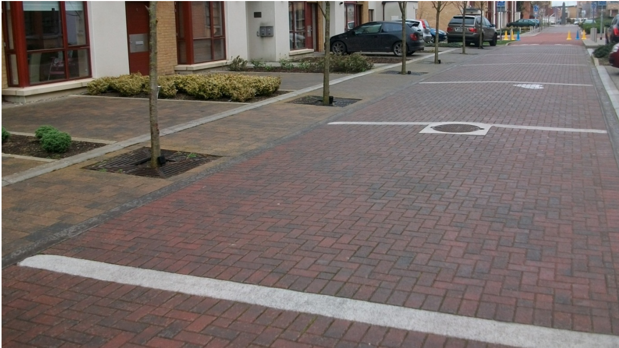
Figure 3.11 – A Shared Surface in Adamstown, Dublin.
