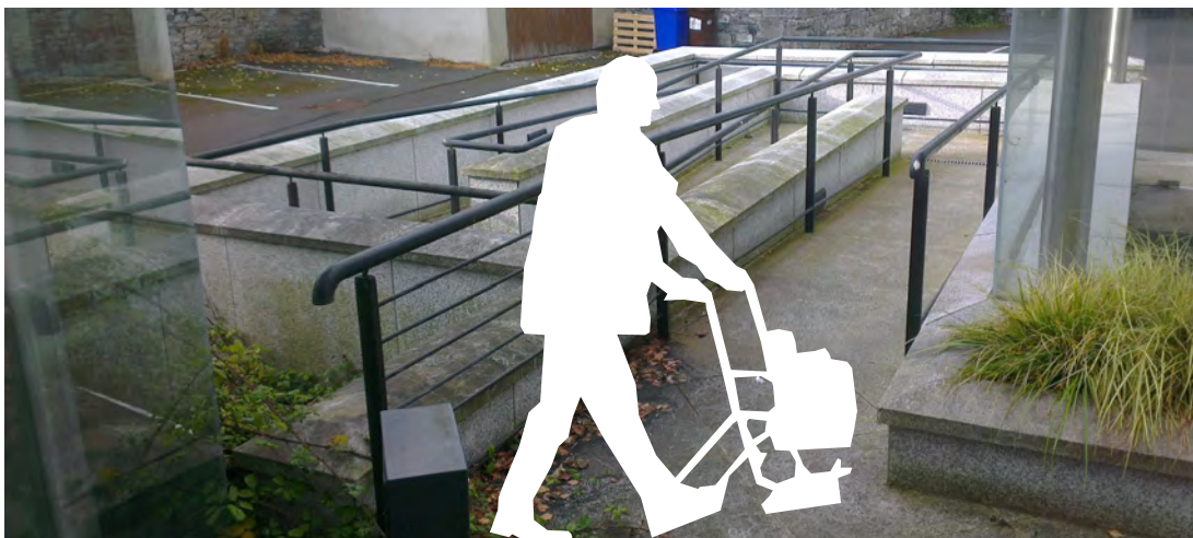
11 Complicated ramp at the main entrance to a building that may be confusing.
