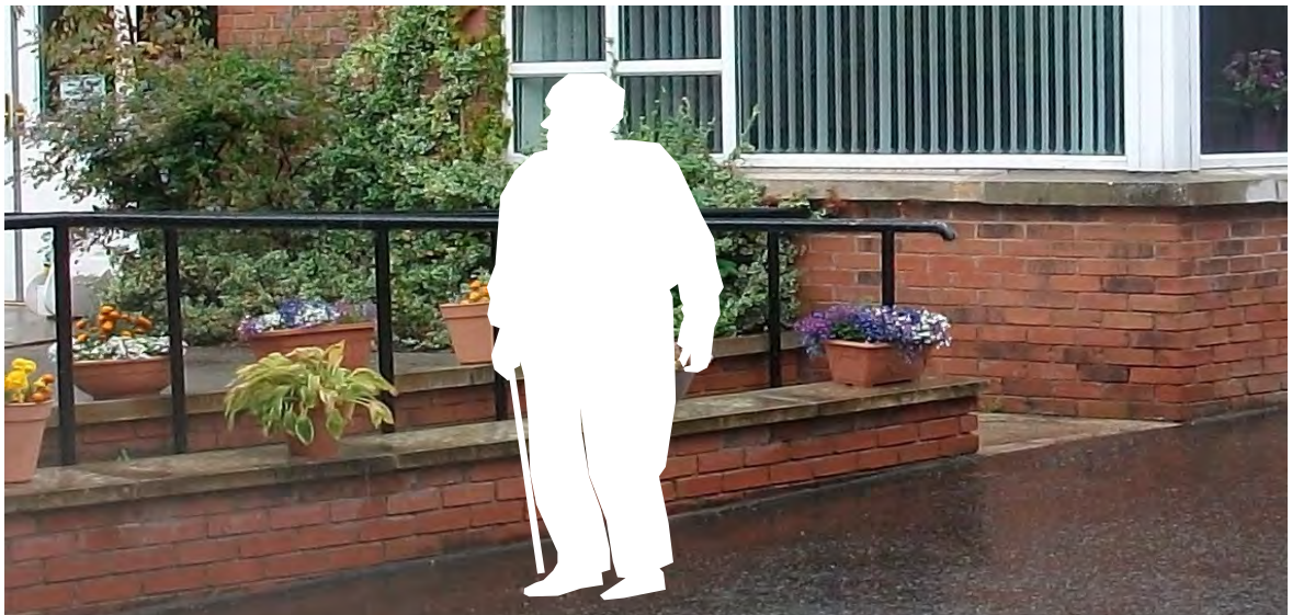
12 Steel handrails to exterior ramp.
