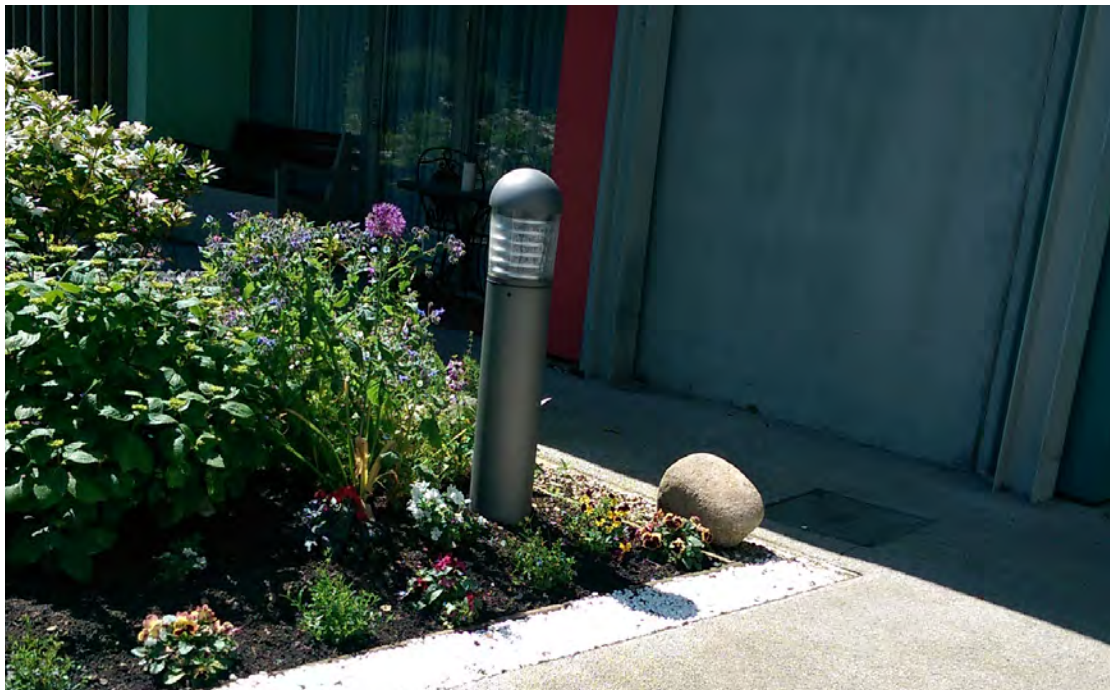
14 Access path with lighting bollard.
