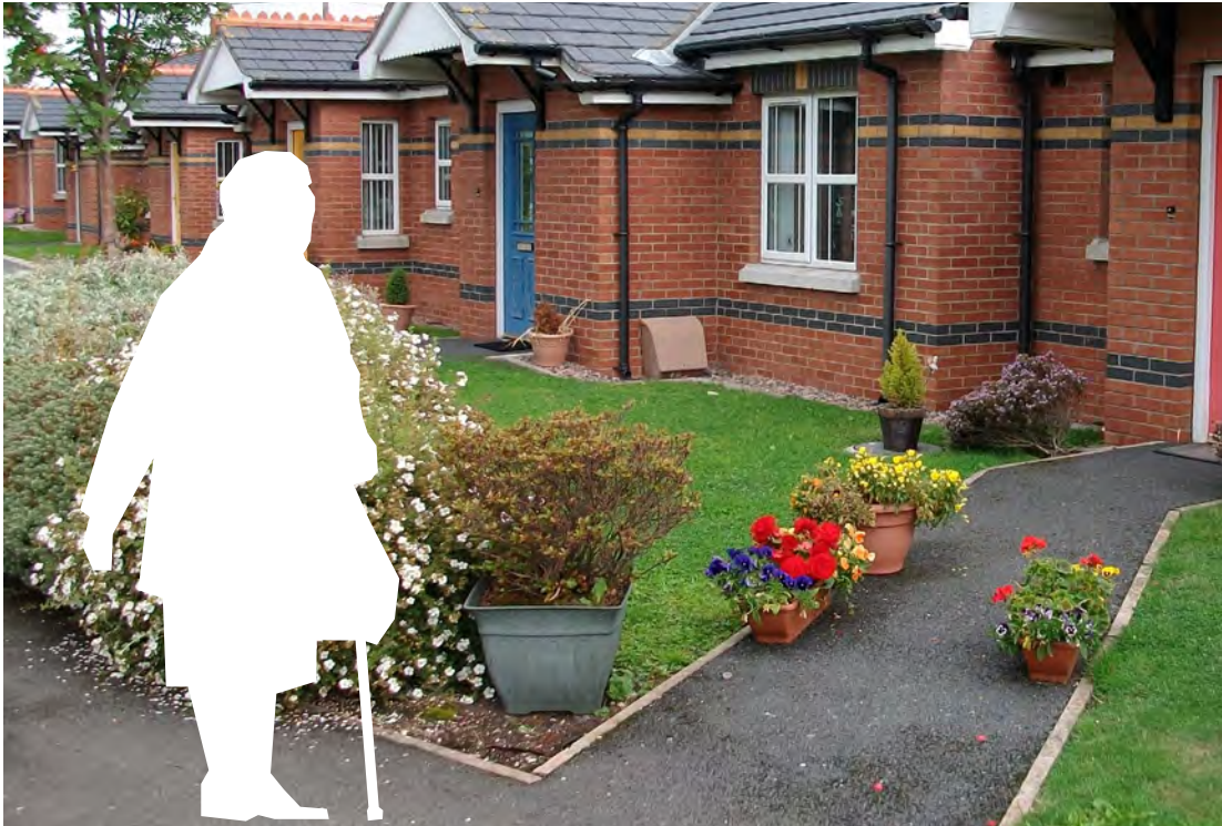
07 The use of painted front doors to create distinctive and identifiable entrances.
