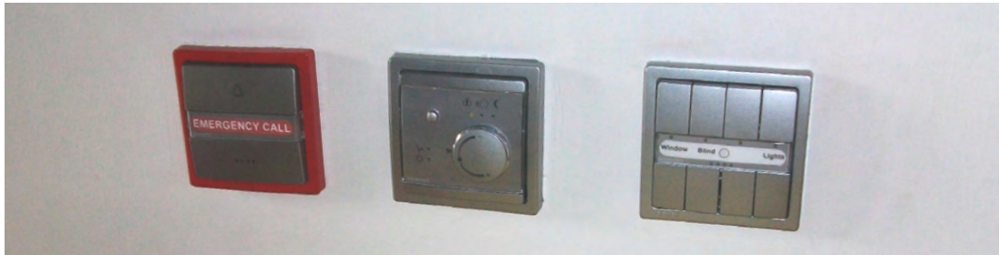
10 Heating controls along with alarm and light switches.
