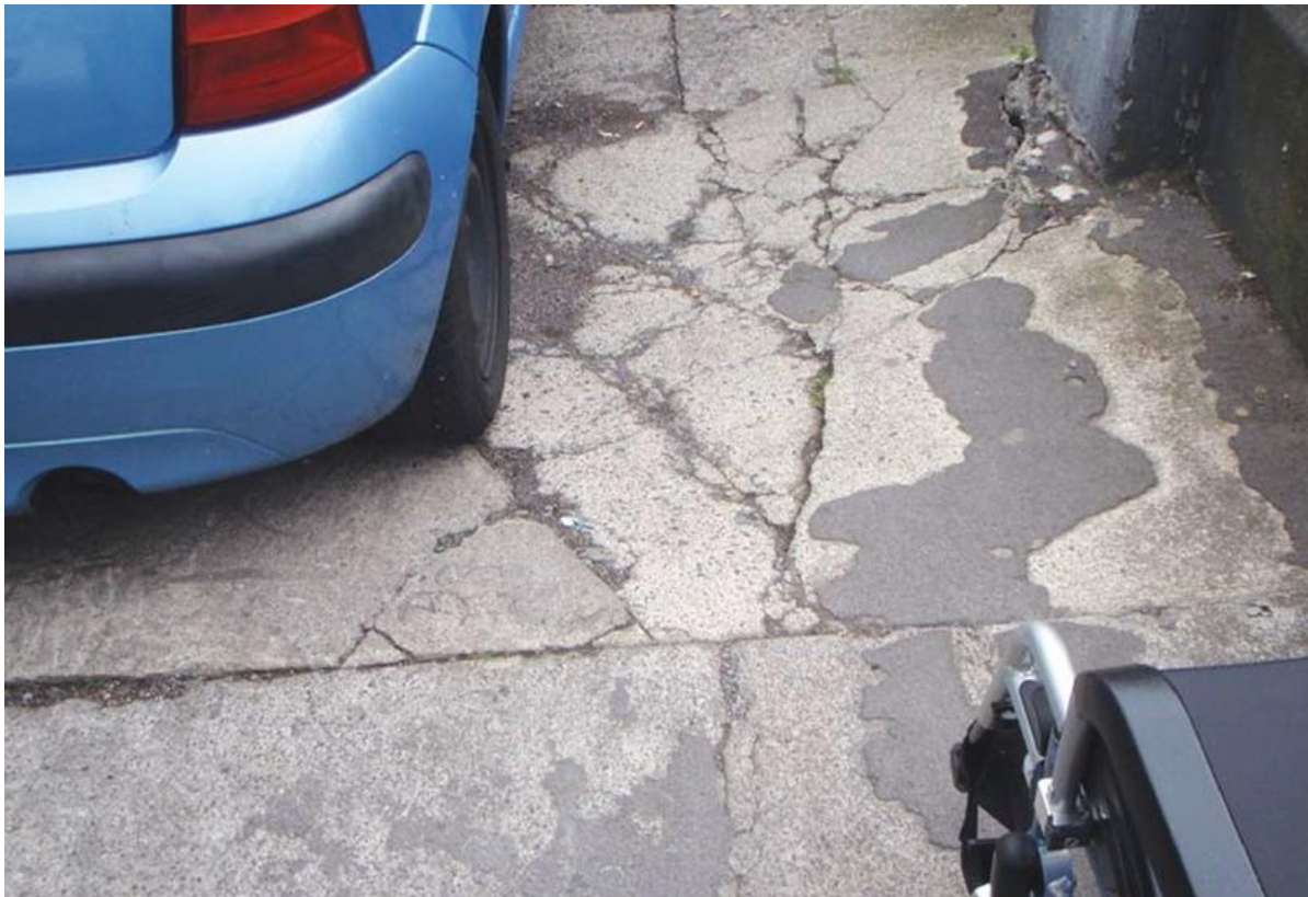
Image 2.2 An example of a car parked on a broken and uneven footpath surface.
